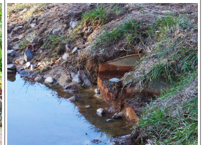
Damaged or clogged inlet and outlet channels, pipes and trash racks. Repair or replace to prevent functionality failure.
