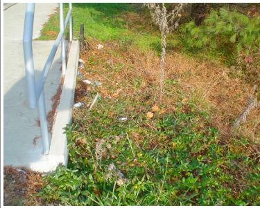
Storm drain obstruction. Remove sediment, debris, and trash to allow flow.
