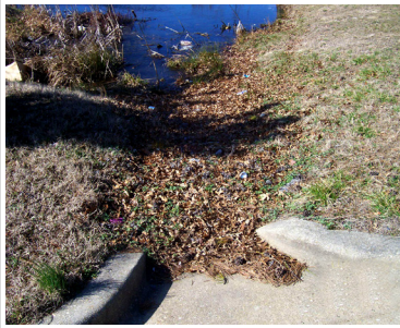
Sediment accumulation at curb opening. Remove sediment and debris to allow water to drain into curb opening.
