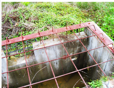
Damaged or corroded trash rack. Repair or replace immediately to prevent clogging and functionality failure.
