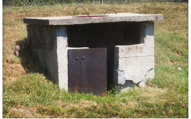
Broken or damaged control structure.
