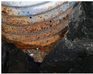
Riser scaling/rusting. Functionality compromised.
