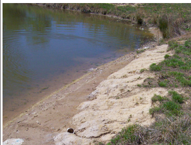
Shoreline erosion on the dam embankment. Address immediately to avoid further erosion.
