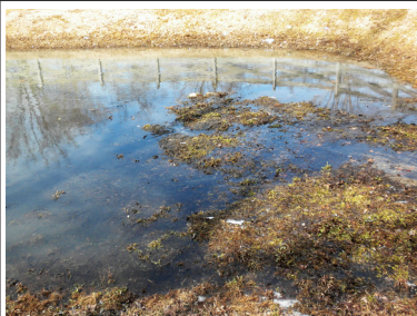
Dry pond holding water longer than 72 hours. Indicates a clog or drainage obstruction.
