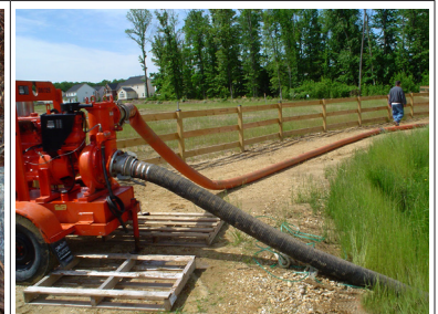
Dredging. Approximately every 10 years ponds should be dredged when the pool volume is half-filled with sediment. Ponds do not effectively remove sediment and pollutants when filled.
