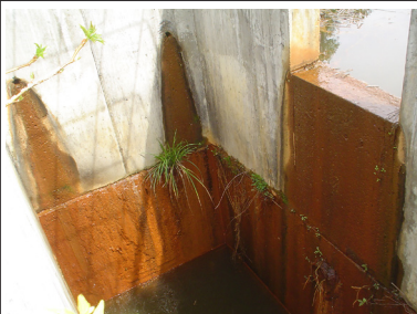
Leaking control structure and pipe joints. Repair or replace immediately to prevent functionality failure.
