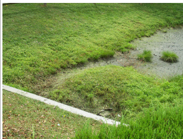
Accumulated sediment and debris in pond. Periodically remove debris from pond water and structures.
