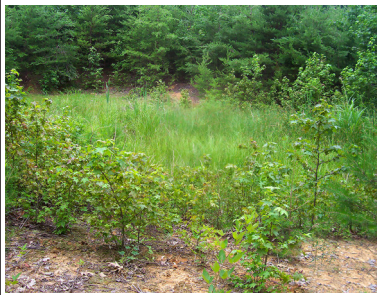
Downstream dam slope not mowed to toe, trees on dam. Can cause dam to collapse.
