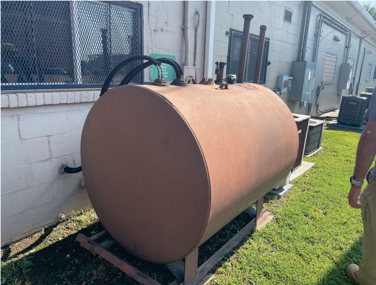
Photograph No. 1 Aboveground storage tank outside of the facility.
