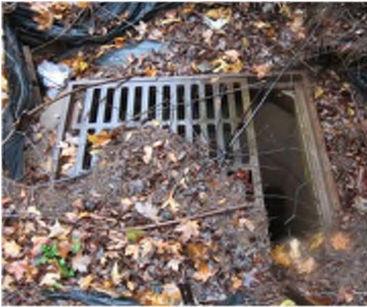
Damaged Grate
