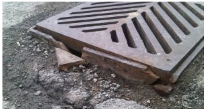
Damaged Frame
