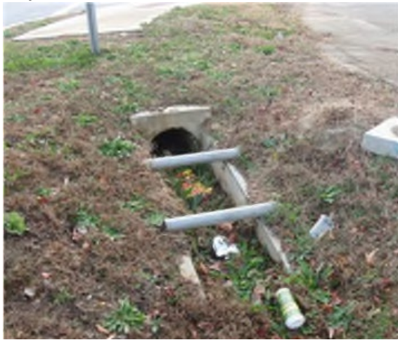
Pipe conveyance filled with vegetation.
