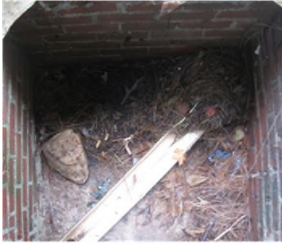
Sediment and debris inside stormwater inlet
