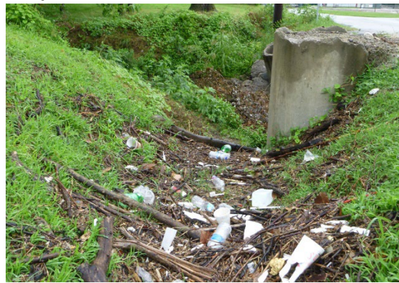
Litter and debris within a swale.
