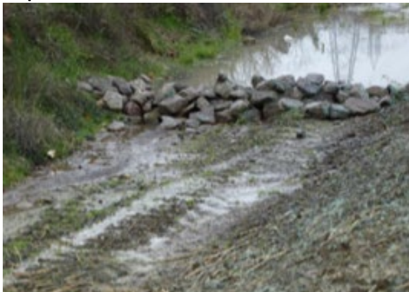
Rock check dam across a channel.
