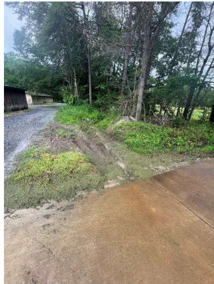
Photograph No. 4 Vehicle wash water drainage ditch.
