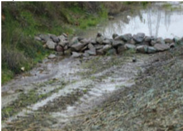
Rock check dam across a channel.
