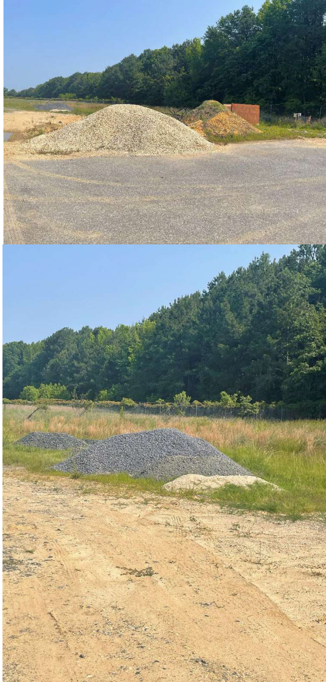
Photograph No. 6 & 7 Stone, gravel, and dirt stockpiles.
