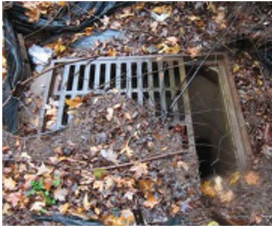
Damaged Grate
