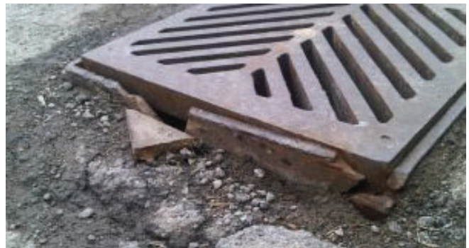
Damaged Frame
