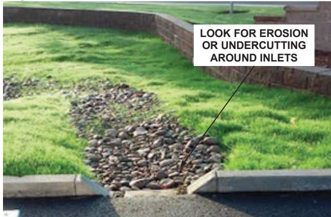
Inlet to a rock-lined swale.
