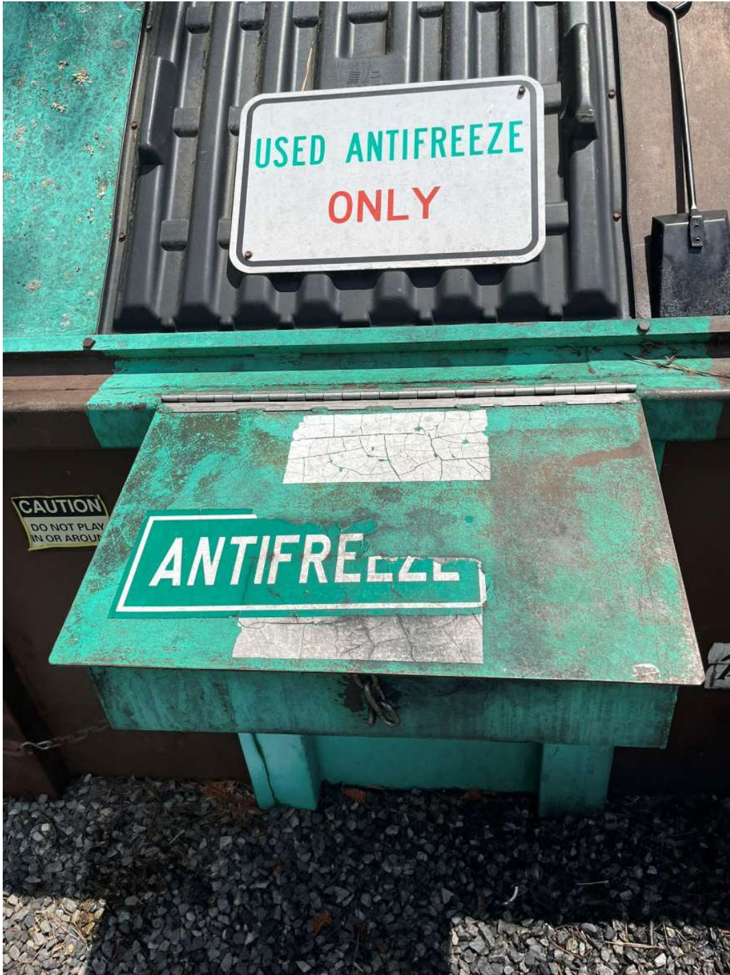
Photograph Nos. 1, 2 & 3 Secondary containment for citizen drop-off for used oil and antifreeze with faded labels.
