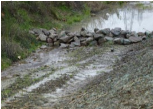
Rock check dam across a channel.
