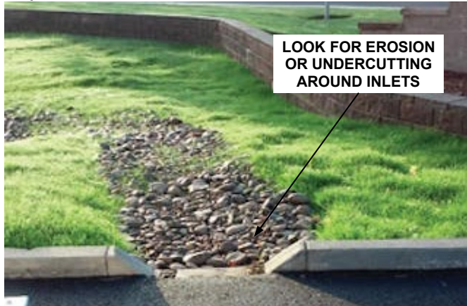
Inlet to a rock-lined swale.
