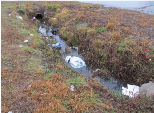
Litter and debris within a ditch.
