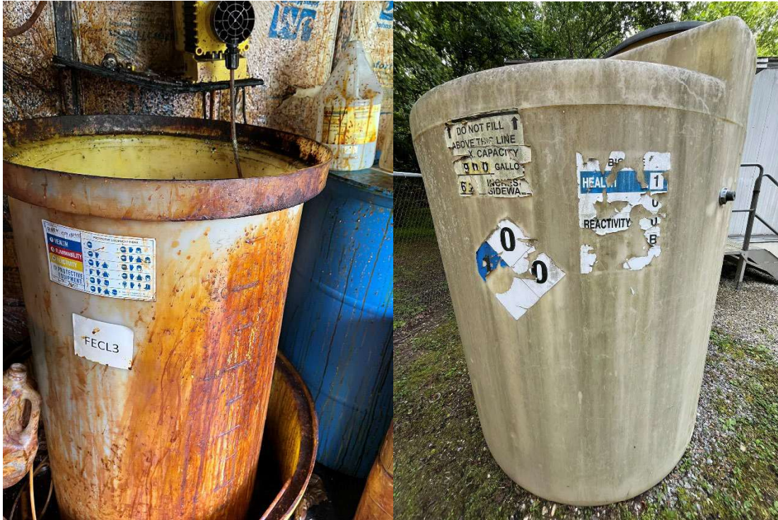
Photograph No. 7 & 8 Storage with labeling needing updating.
