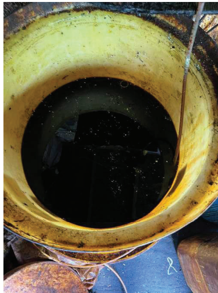
Photograph No. 9 Ferric chloride storage photo.
