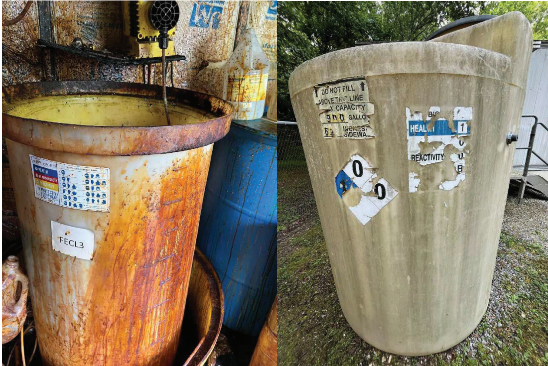
Photograph No. 7 & 8 Storage with labeling needing updating.
