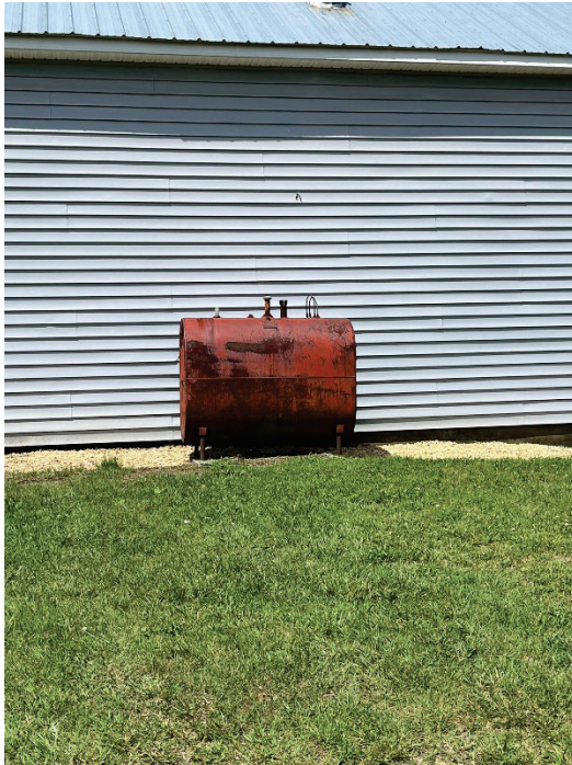
Photograph No. 1 & 2 275-gal AST, contents assumed #2 heating oil.
