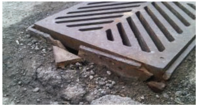
Damaged Frame
