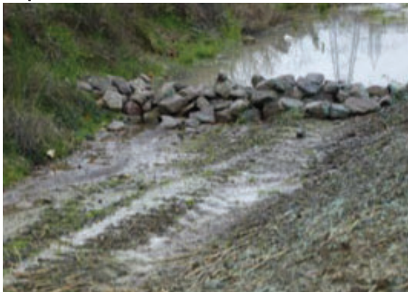
Rock check dam across a channel.
