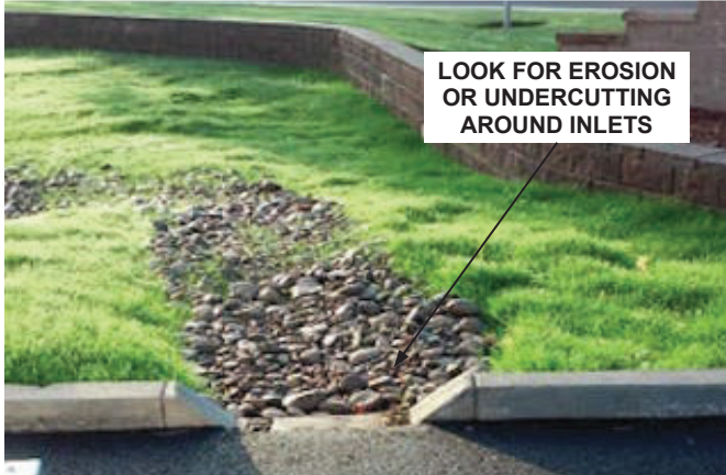
Inlet to a rock-lined swale.
