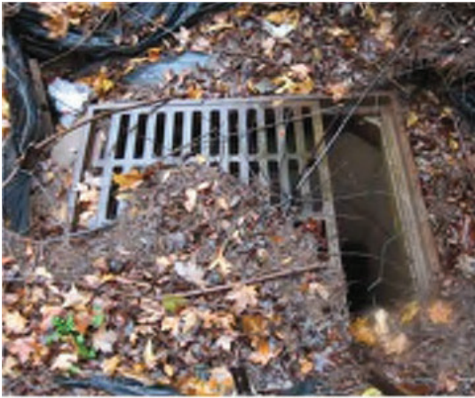
Damaged Grate
