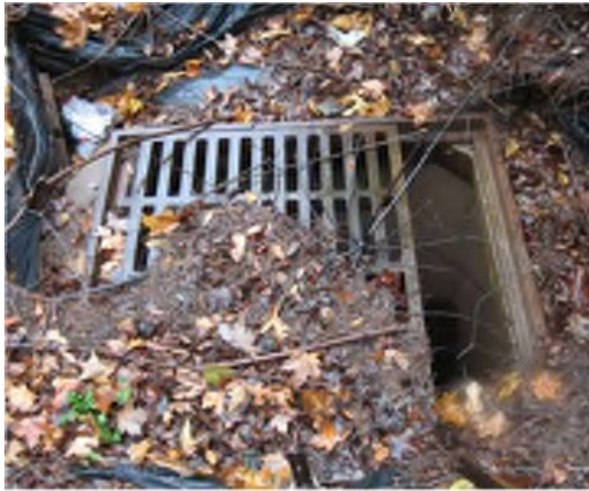
Damaged Grate
