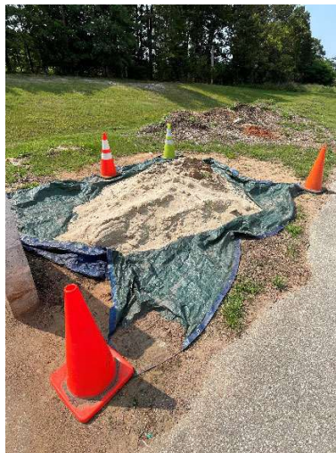
Photograph No. 9 Sand stockpile next to other stockpile bays.
