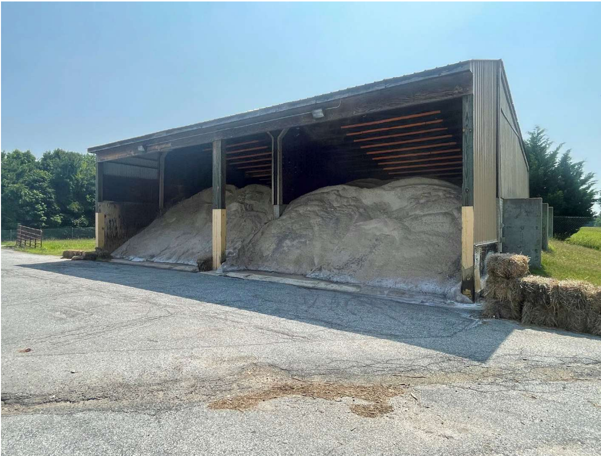
Photograph No. 13 Salt barn on site with haybales placed to the side.
