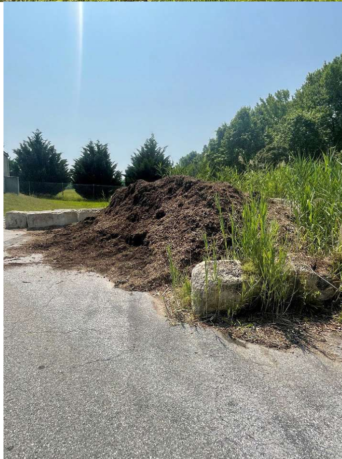
Photograph Nos. 9, 10, 11, & 12 Stockpiles of mulch, gravel, and aggregate materials at risk of stormwater runoff.
