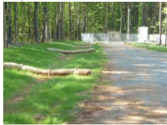
Filter sock check dams across a grass swale.
