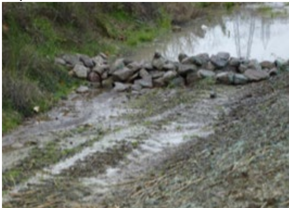
Rock check dam across a channel.
