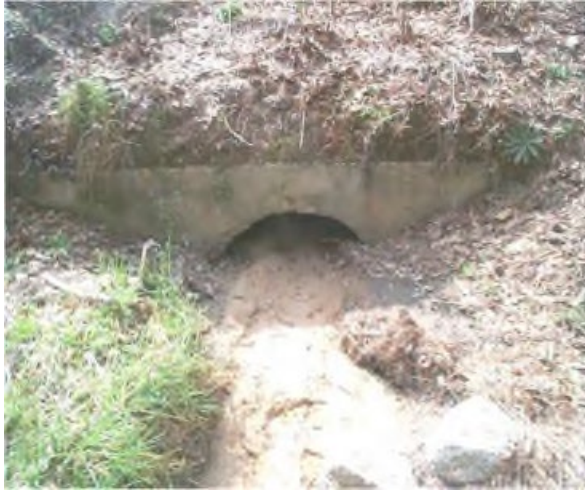
A pipe filled with sediment, inhibiting flow.
