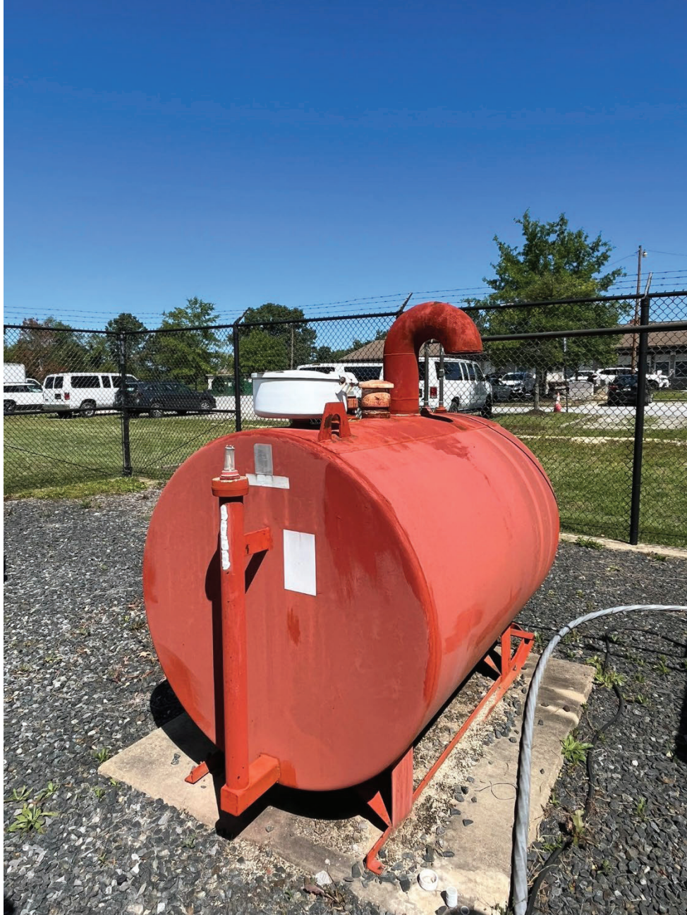
Photograph No. 2 Aboveground storage tank outside of facility with faded labels.
