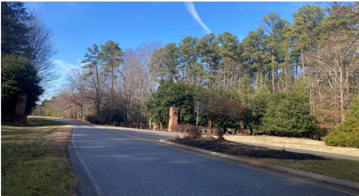
Figure 5 - Swan Point Road at the entrance gateway to the Swan Point subdivision – this roadway has no paved shoulders. As is, this roadway does not accommodate pedestrian and bicycle use.
